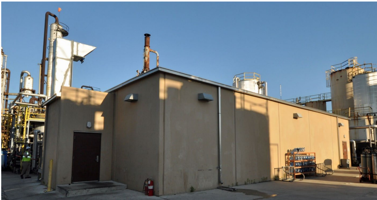
Figure 5. Reaction Control Room. KMCO’s blast-resistant control room. (Credit: CSB)
