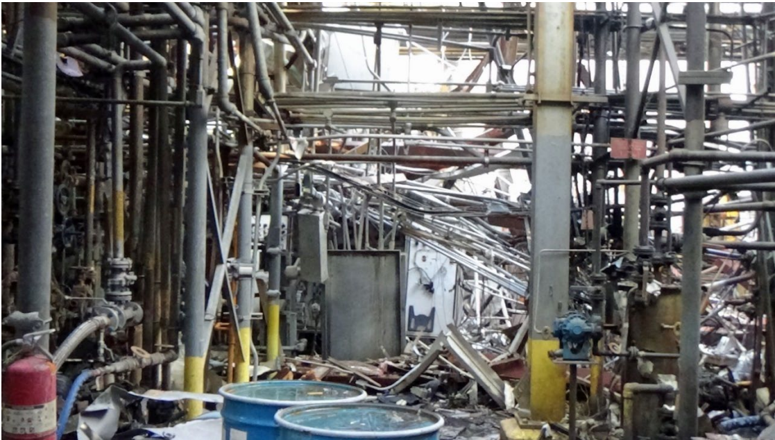
Figure 13. R2 Building (North Side). This post-incident photo shows the path KMCO workers commonly took to enter the R2 Building. With process units on the left and right, this walkway led to the entrance on the north side of the R2 Building, where emergency responders found Board Operator 2. (Credit: CSB)
