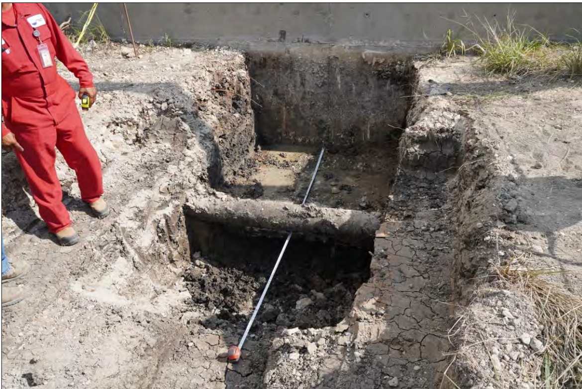
Photo 22: Containment wall footing excavation, south face of north wall, inside containment area
