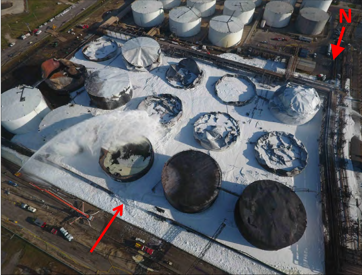
Photo 4: Containment wall failure (red arrow) during fire suppression efforts 12
