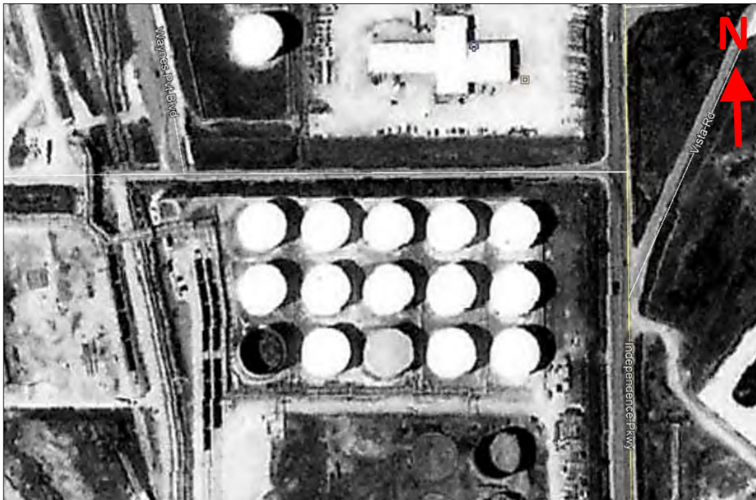
Photo 2: Aerial photo of first & second 80's tank farm, 1978
