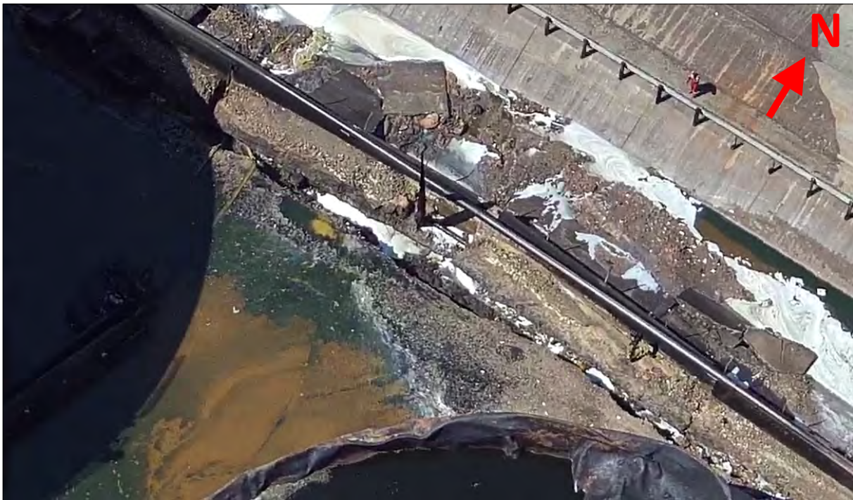
Photo 7: Aerial photo of containment wall failure after water flow stopped and before temporary dike wall was constructed 15
