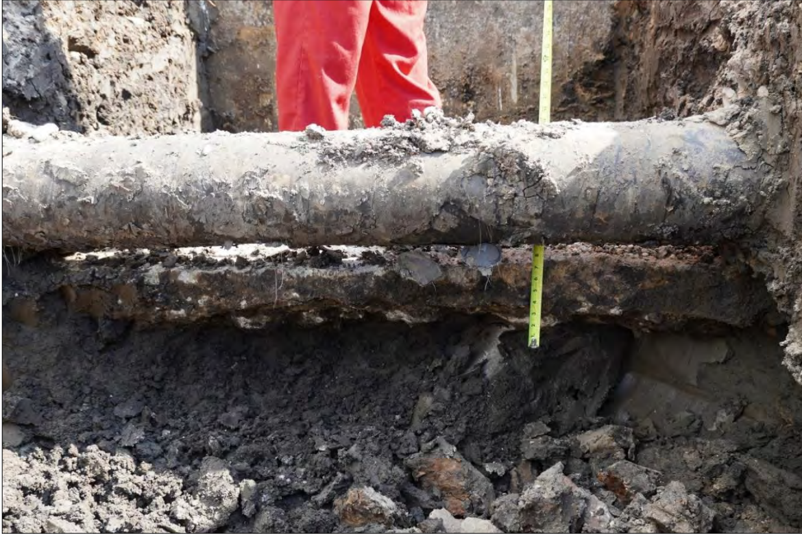
Photo 23: Containment wall footing and underside of footing
