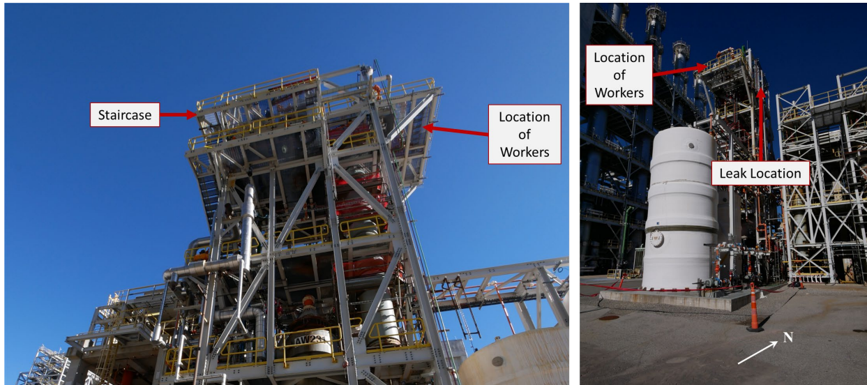
Figure 11. Location of trapped workers. When the release occurred, two Jake Marshall employees and four Pen Gulf employees were working on the south end of the platform. Directional arrow is approximate. (Credit: CSB)
