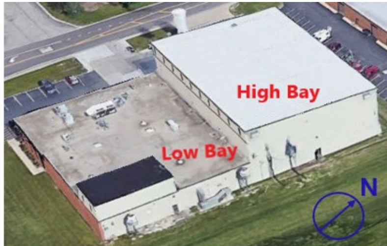
Figure 2. AB Specialty production building. (Credit: Google Maps with annotations by CSB)
