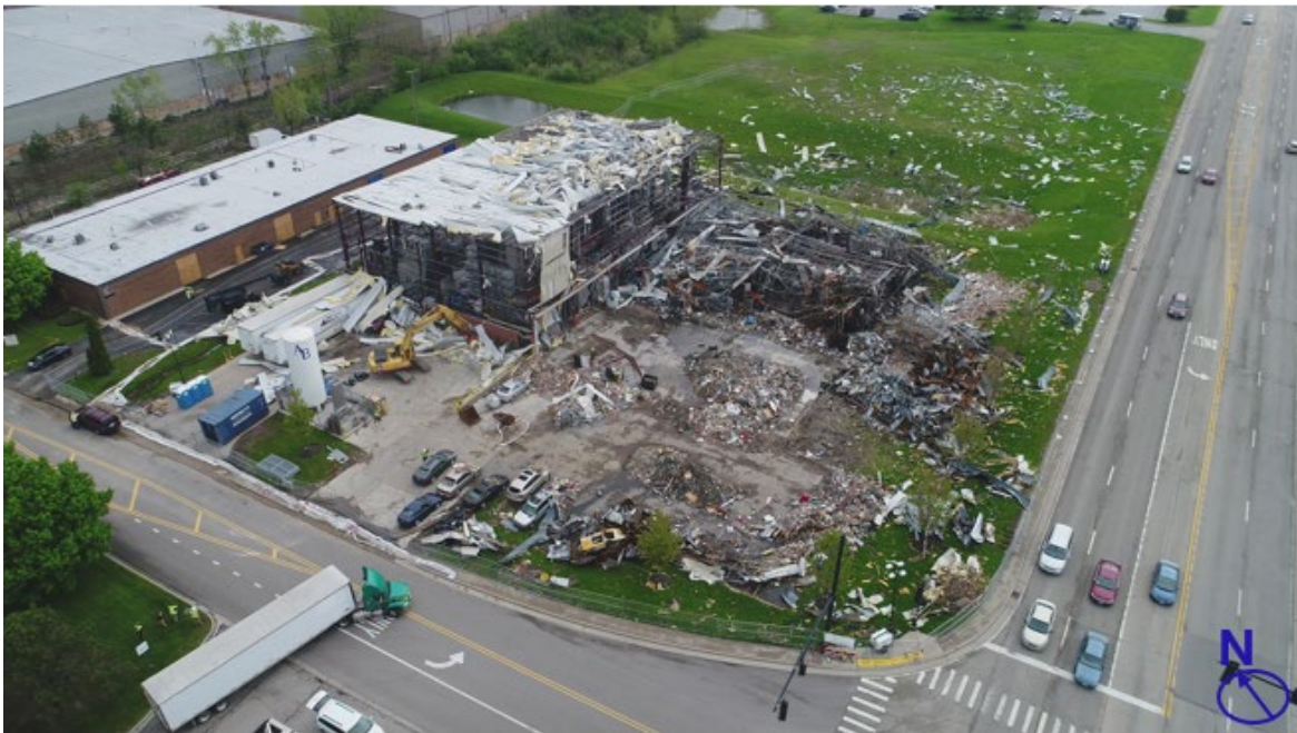
Figure 12. Post-explosion photo of the AB Specialty facility. (Credit: CSB)
