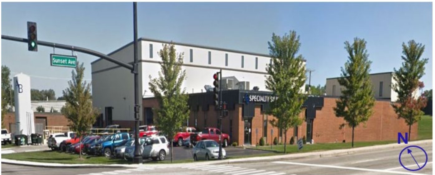
Figure 1. AB Specialty production facility in Waukegan, Illinois, before the incident. (Credit: Google Earth)
