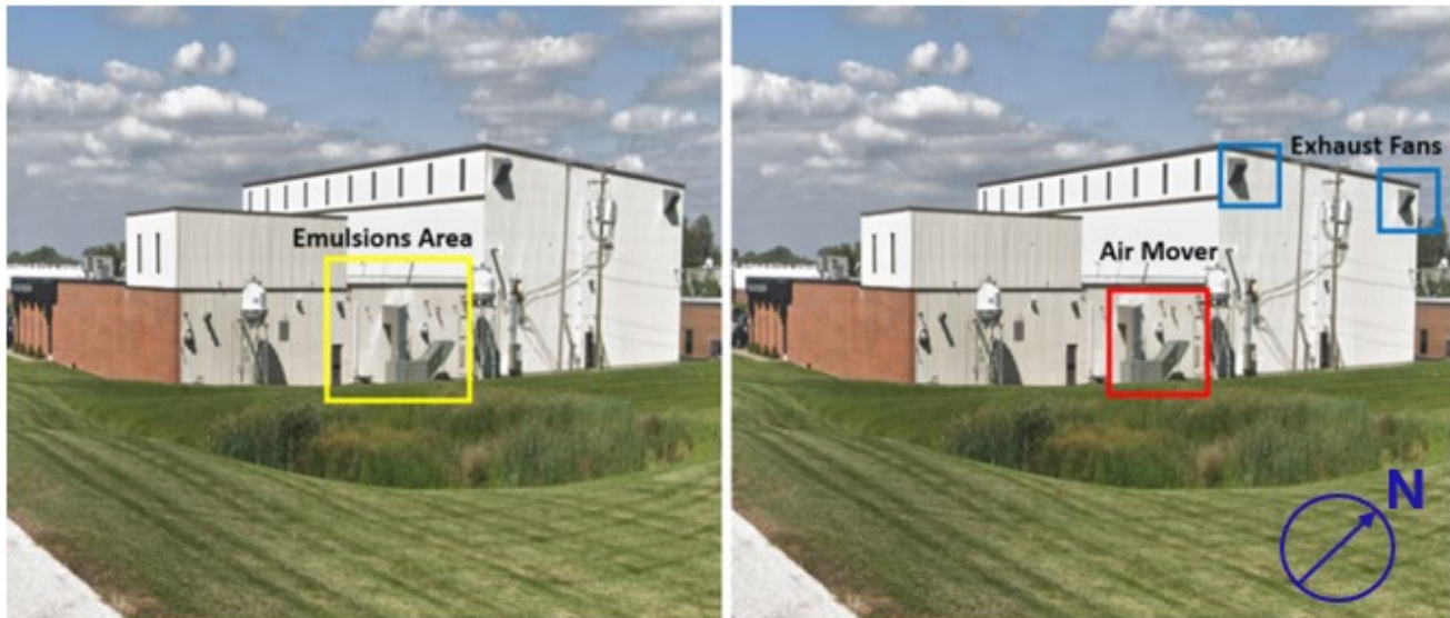
Figure 6. Location of the emulsions area and the ventilation system components. (Credit: Google Maps with annotations by CSB)
