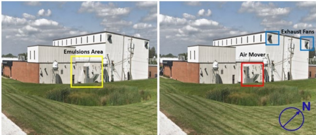
Figure 6. Location of the emulsions area and the ventilation system components. (Credit: Google Maps with annotations by CSB)
