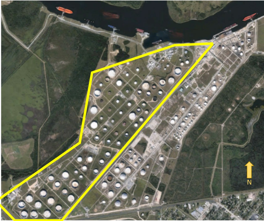
Figure 1. Overhead view of Nederland terminal. (Credit: Google Earth; Adapted by CSB)
