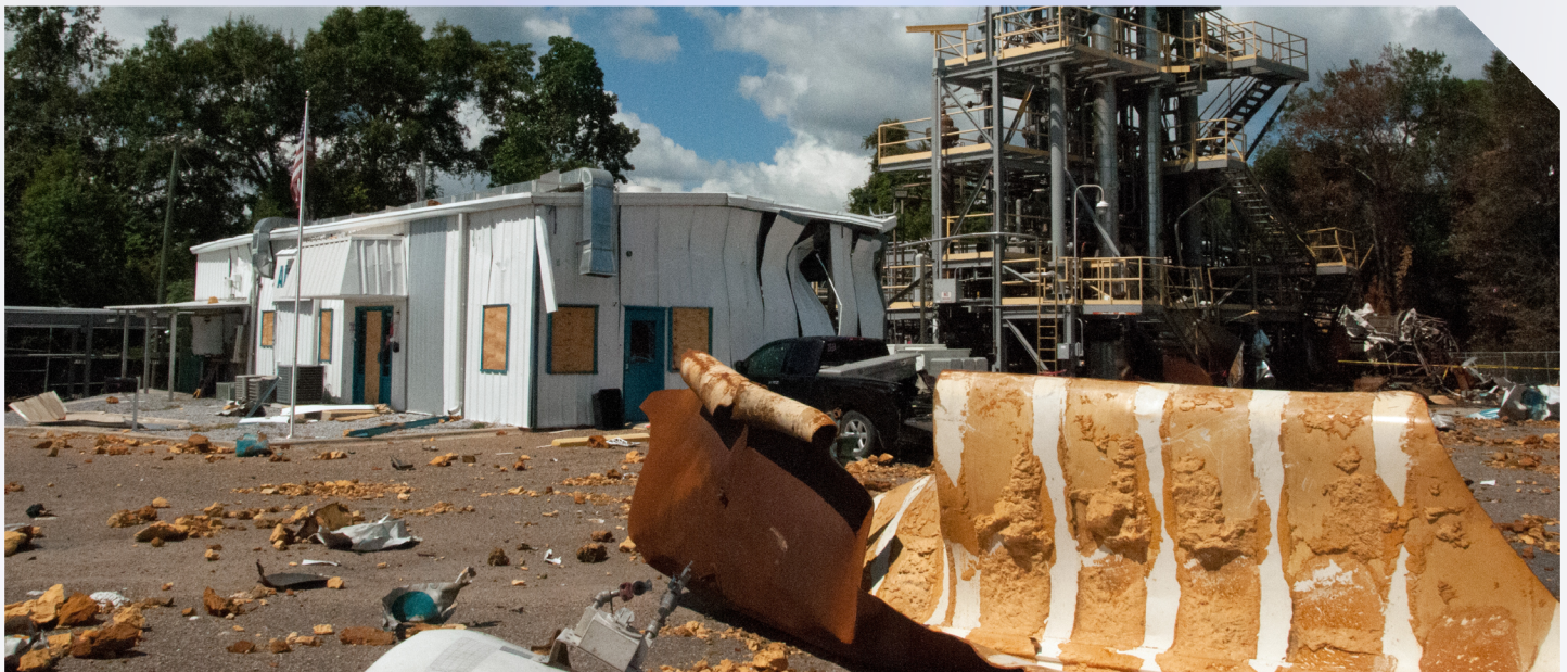
Post-incident photo of the administrative and operations building at the Airgas nitrous oxide manufacturing facility in Cantonment, Florida nitrous oxide manufacturing facility.
