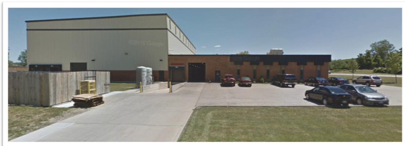
Figure 1. AB Specialty Silicones. Photo showing the AB Specialty Silicones production area (3790 Sunset Ave.) in Waukegan, IL, before the explosion. (Source: Google Maps).
