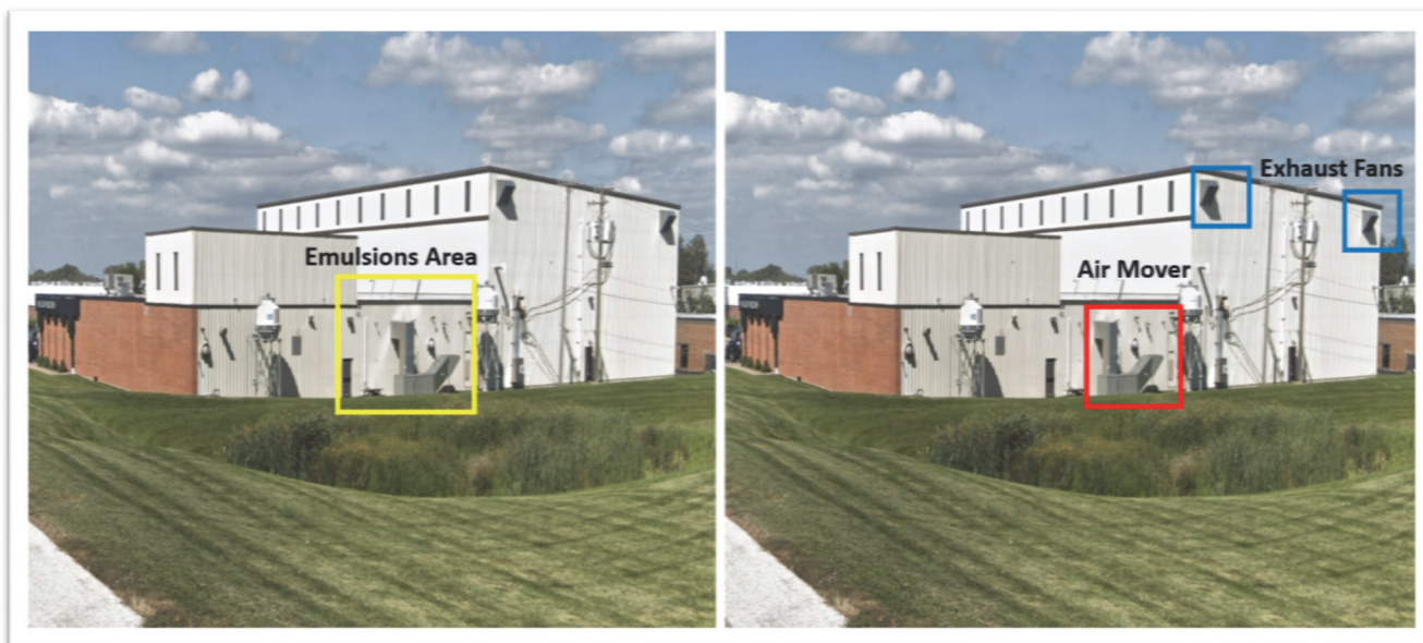
Figure 4. Location of the Emulsions Area and the Ventilation System on the East Side of the Building. Photo on the left shows where the Emulsions Area (yellow box) is located. Photo on the right shows the location of the Air Mover in the Emulsions Area (red box) and the Exhaust Fans in the High Bay (blue boxes). (Source: Google Maps with annotations by CSB).
