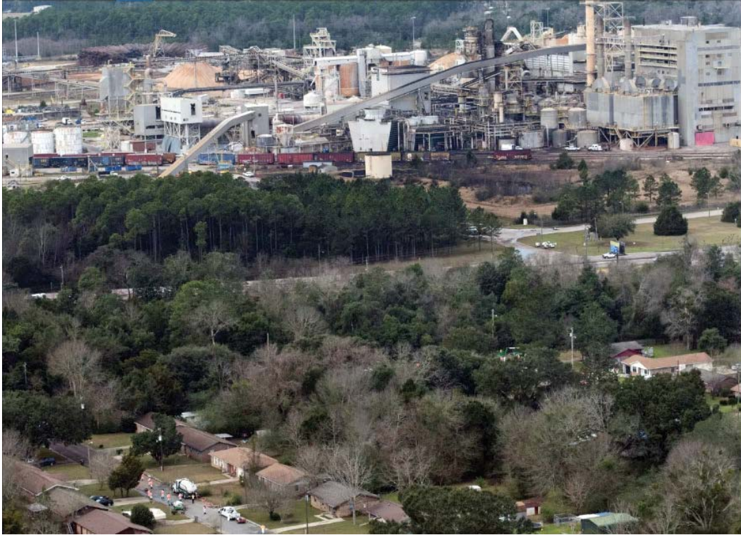
Figure 41. Post-Incident Photograph of the International Paper Pensacola Mill in Relation to Adjacent Neighborhoods. Clean-up crews can be seen in the neighborhood at the bottom left of the photograph. Photograph: Pensacola News Journal [48].
