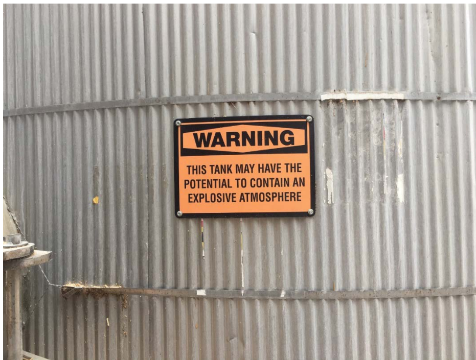
Figure 44. Post-Incident Warning Label. This warning label is intended to inform personnel of the potential hazards associated with a flammable atmosphere inside a vessel. Photograph: PCA.
