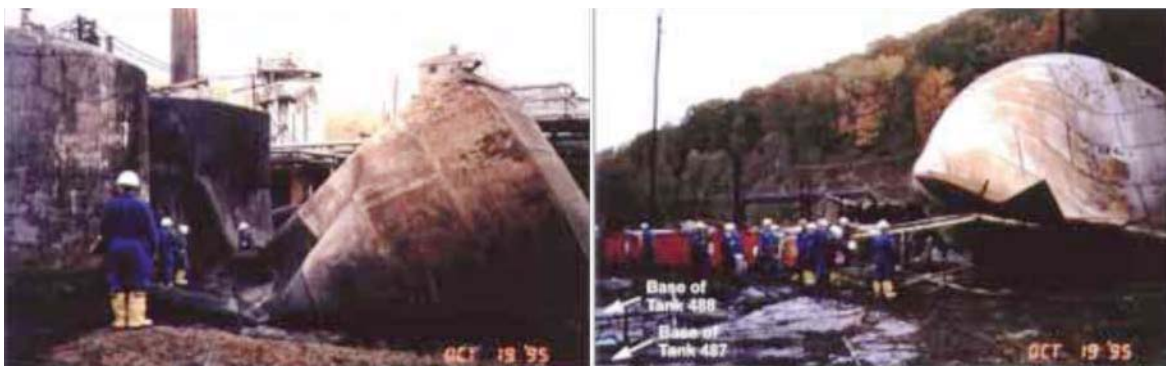
Figure 38. Photographs from the Pennzoil Refinery. These post-incident photographs show the October 1995 explosion at the Pennzoil refinery in Rouseville, Pennsylvania. Photograph credit: [43].
