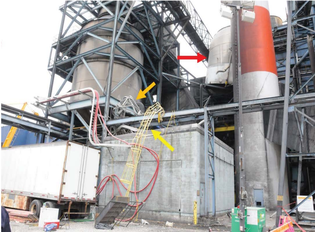
Figure 9. Post-Incident Photograph Showing the Location of the Foul Condensate Tank and Associated Structures. The foul condensate tank is indicated by the red arrow. The ladder previously attached to the tank is indicated by the yellow arrow. The pipe rack, which had previously been located above the tank, is indicated by the orange arrow. Photograph: CSB.
