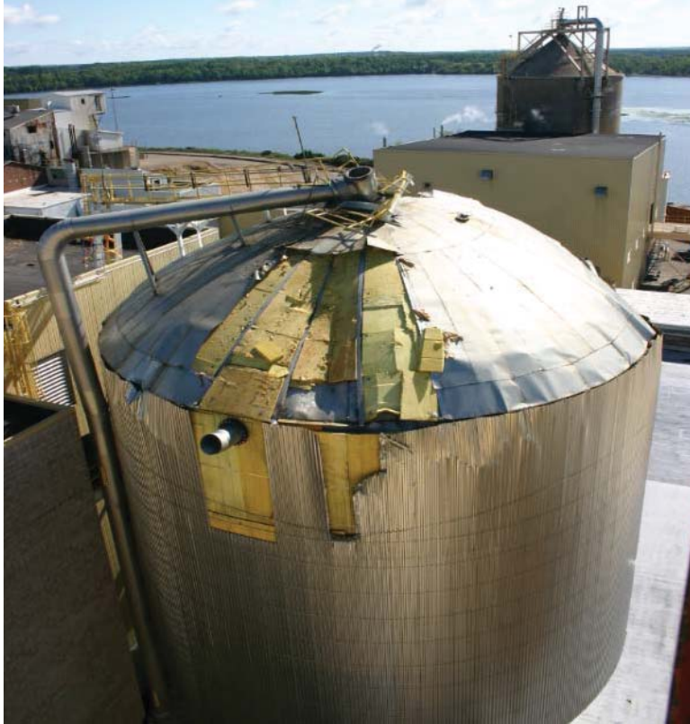
Figure 39. Post-Incident Photograph at the PCA Tomahawk Mill. This photograph shows the post-incident storage tank at the PCA Tomahawk mill in 2008. Photograph: CSB.
