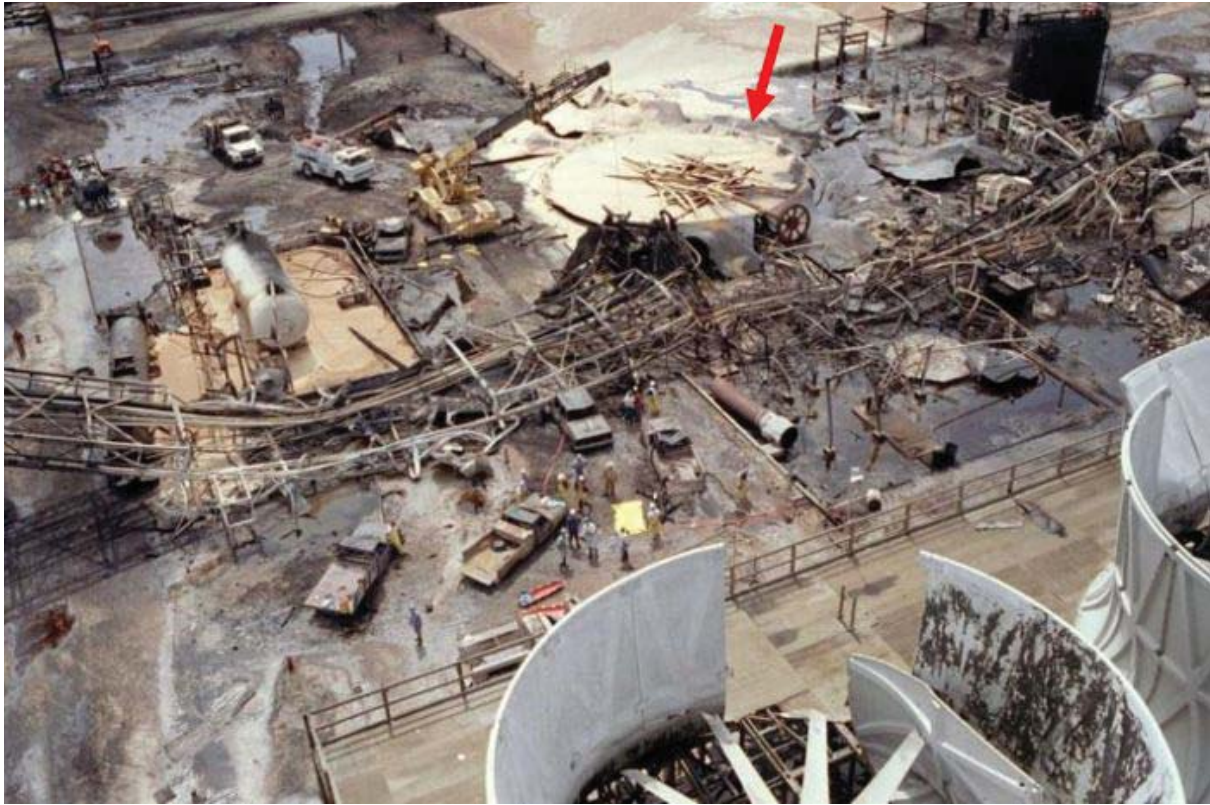
Figure 36. Post-Incident Photograph of the July 1990 Explosion at the ARCO Chemical Facility in Channelview, Texas. The location of the wastewater storage tank is indicated by the red arrow. Photograph credit: [41].
