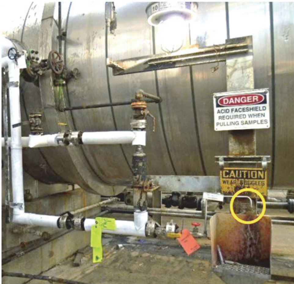
Figure 11. Photo of the sulfuric acid sample station at the Company Y refinery. The photo shows a typical sulfuric acid sampling station at the refinery. The yellow circle identifies the location where the operator obtains the acid sample.
