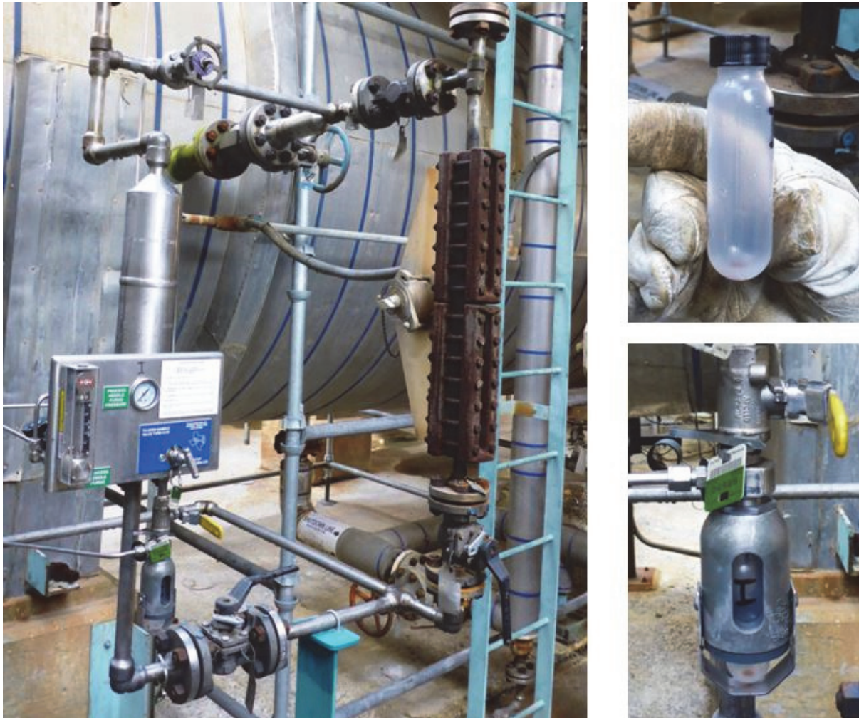
Figure 10. Photo of the sulfuric acid sample station at the Company X refinery. The photo on the left shows a typical sample station used by Company X workers to obtain sulfuric acid samples. The photo on the top right shows a typical sample bottle and the photo on the bottom right shows the sample bottle installed to obtain a sample.
