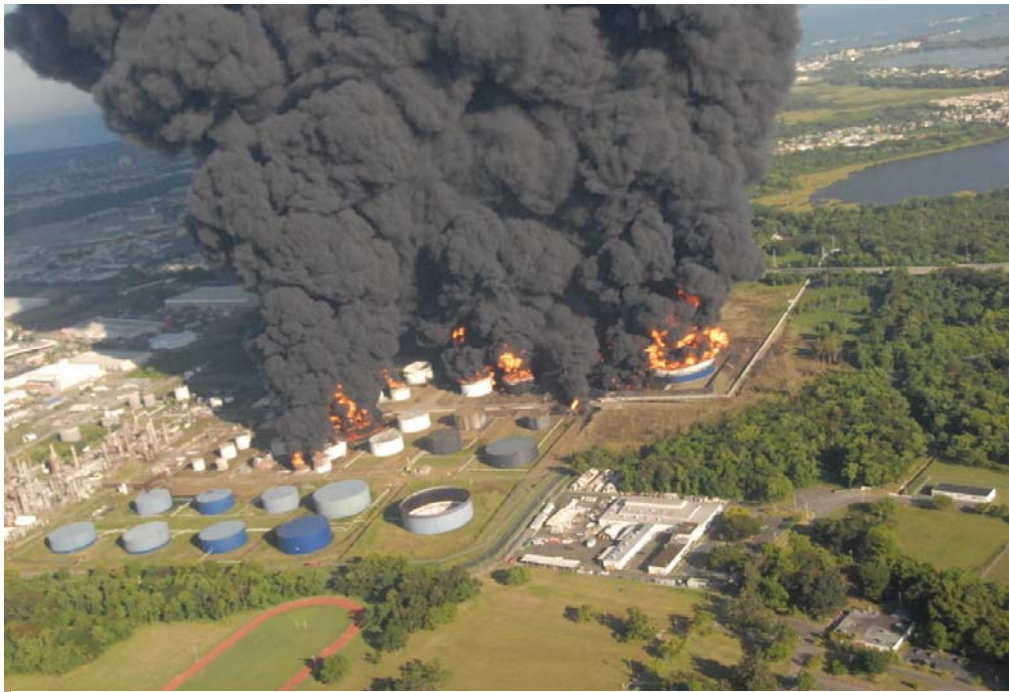
Figure 5: CAPECO multiple tank farm fire, October 23, 2009.
