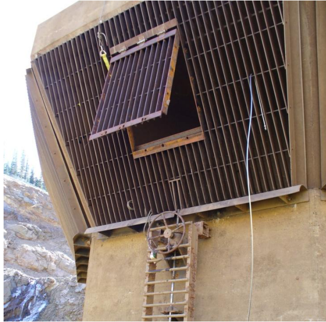
Figure 3. Upper reservoir mushroom access hatch
