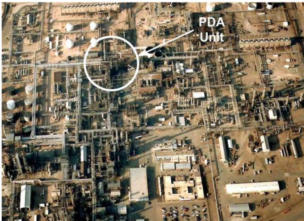
Figure 1. PDA unit location in the McKee Refinery
