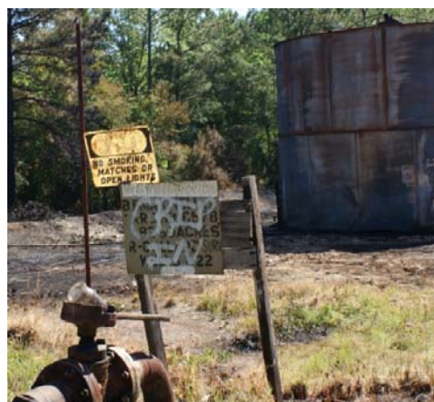
Figure 6-10: M-C Production tank site with warning sign
