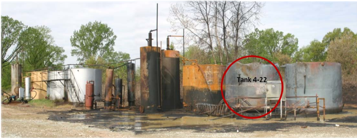
Figure 6-6: Weleetka, OK, oil and gas well site indicating Tank 4-22, which exploded
