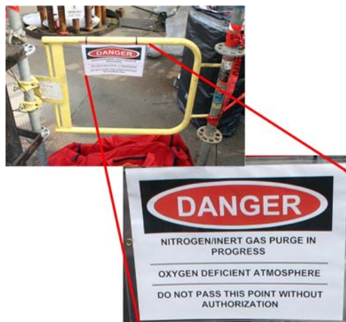
Figure 8. Nitrogen-purge controlled area barricade and warning installed on the R1 platform after the incident.
