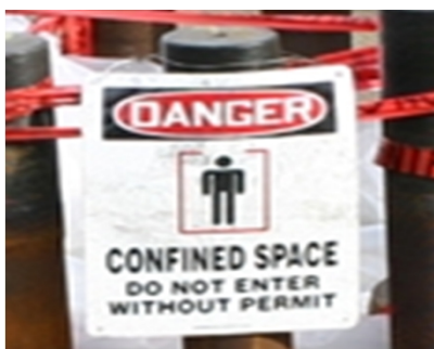
Figure 10. Typical sign used to identify unsecured confined space access opening.
