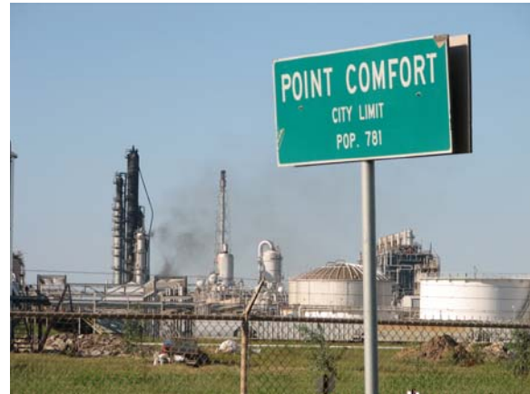
Figure 2. View of the Damaged Plant from Highway 35.
