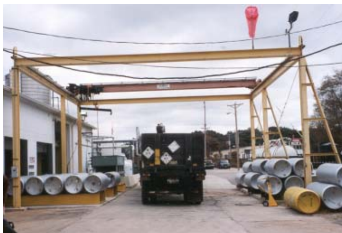
Figure 26. Truck loading station at DPC Festus.
