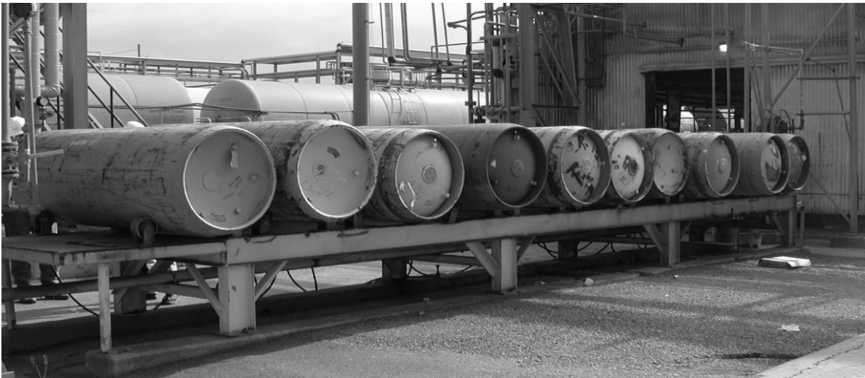
Figure 12. 1-ton refrigerant cylinder prep rack.
