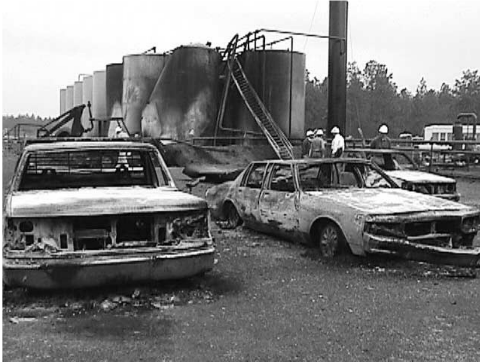
Figure 7. Damaged Vehicles and Storage Tanks
