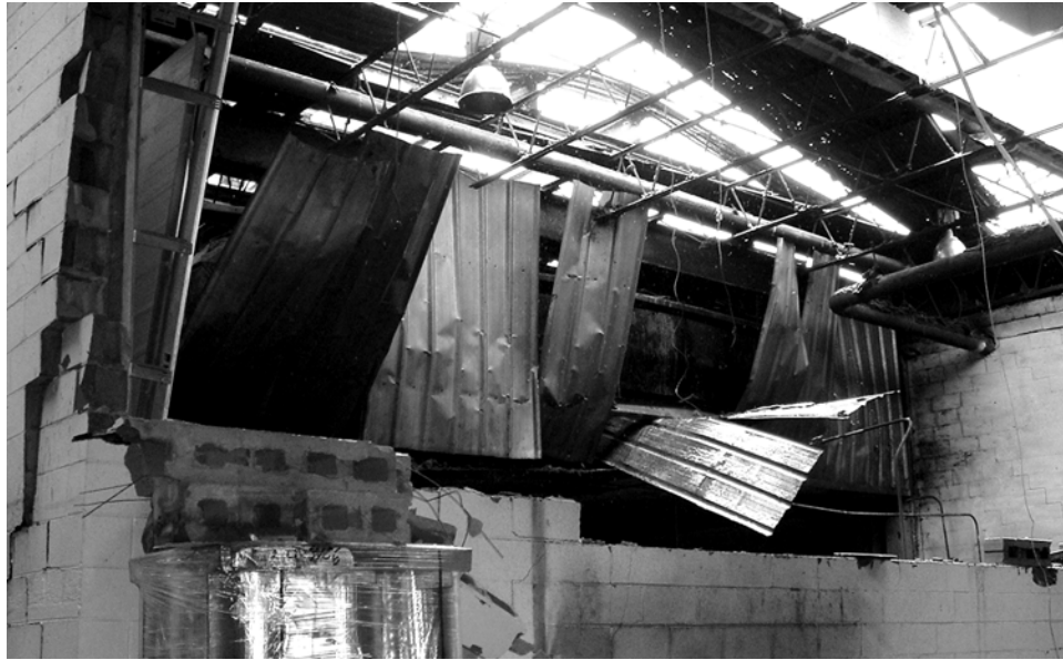
Figure 6. Collapsed firewall and metal panels at south end of line 405 blend room.
