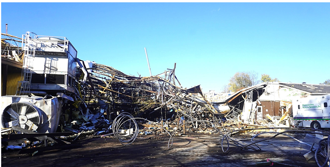
Figure 5. Property damage at the Givaudan facility in Louisville, Kentucky. (Credit: CSB)
