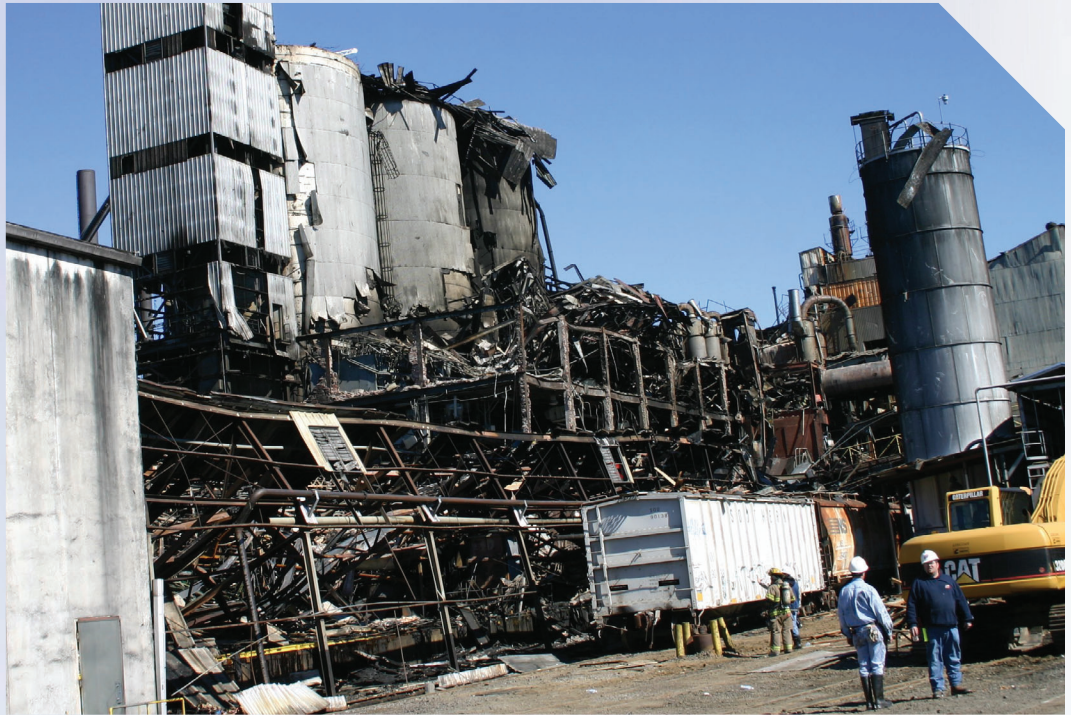
View of the massive damage caused by the combustible dust explosions and fires at Imperial Sugar.
