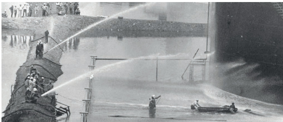
Figure 2. Image of firefighters working to close valve on storage tank. Courtesy of the Special Collections Research Center. Temple University Libraries. Philadelphia, PA.
