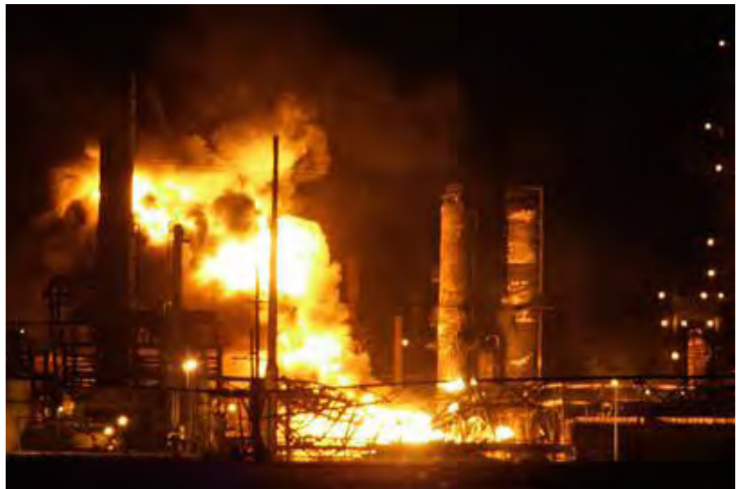
Figure 5. Photos included in the CSB Valero McKee Investigation Report. This photo is courtesy of the Associated Press.
