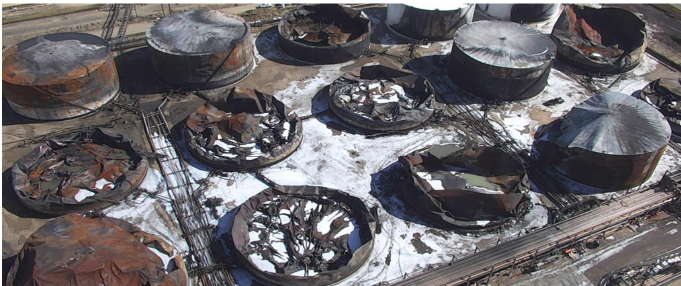
Figure 8. Photo included in the CSB ITC Investigation Report. This photo shows an overhead view of the First & Second 80's tank farm containment wall failure that allowed materials to enter the surrounding waterways on Friday, March 22, 2019. (Credit: ITC).
