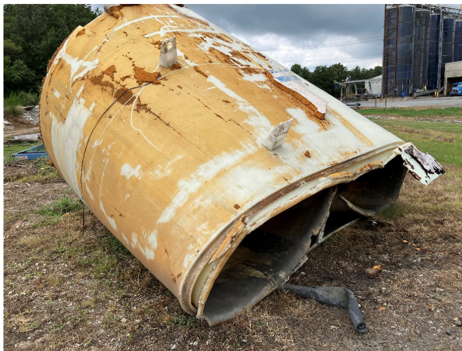
Figure 1. Ruptured Polyethylene Tank at Darling. (Credit: Darling)
