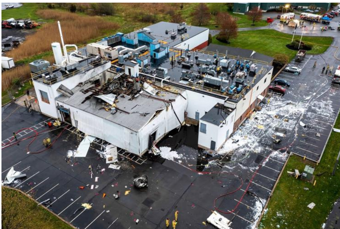
Figure 1. Damages After Explosion at PCI. (Credit: The Salem News)
