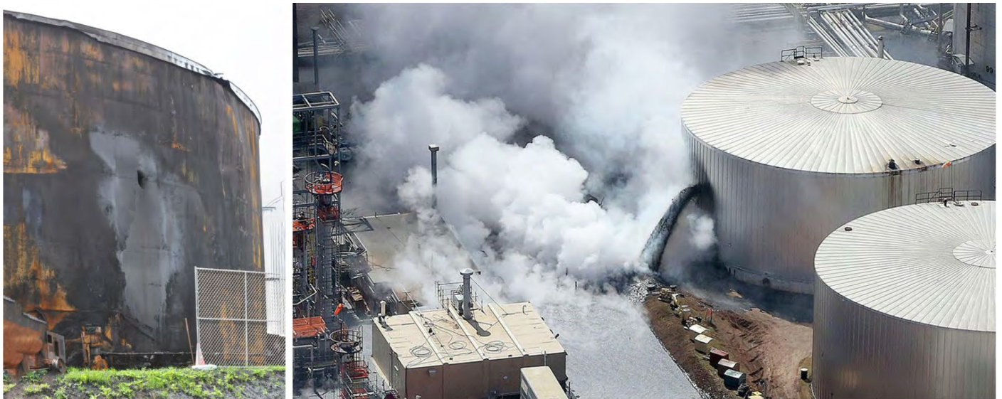
Figure 33. Post-incident photographs of the leaking asphalt storage tank at the Husky Superior Refinery. (Left photo credit: CSB. Right photo credit: Duluth News Tribune [50])
