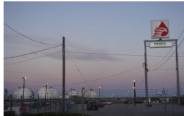
Figure 1. PEMEX Deer Park Refinery (Credit: CSB)
