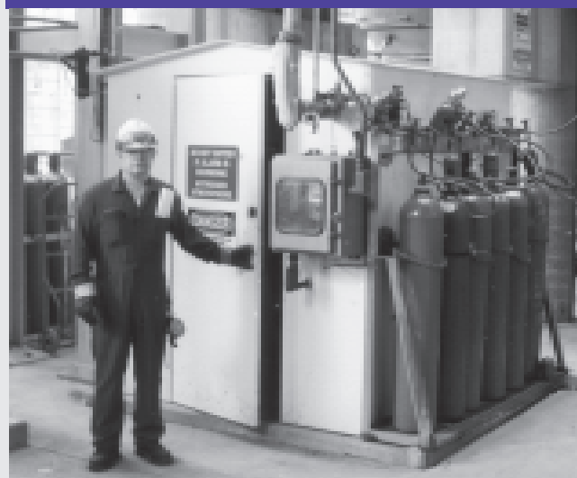
• • Figure 2. Confined area.
