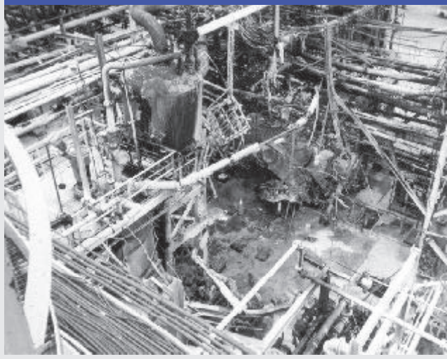
● Figure 3. Site of ruptured reactor, CONDEA Vista Company detergent alkylate plant.
