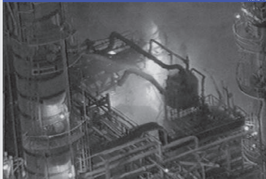
● Figure 4. CONDEA Vista plant fire.
