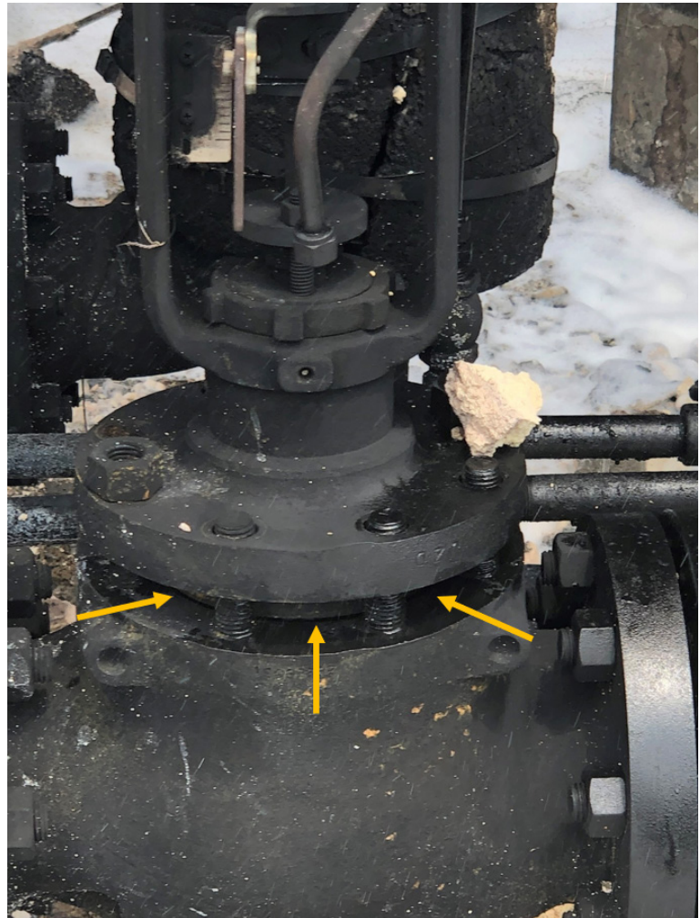
Figure 2. Naphtha release point (gold arrows). (Credit: CVR Energy with annotations by CSB)
