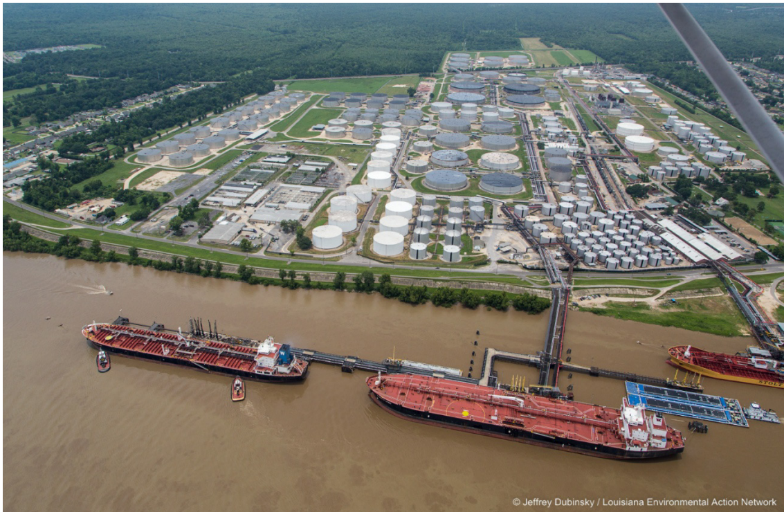
Figure 12. The IMTT facility in St. Rose, Louisiana. (Credit: Jeffrey Dubinsky / Louisiana Environmental Action Network)
