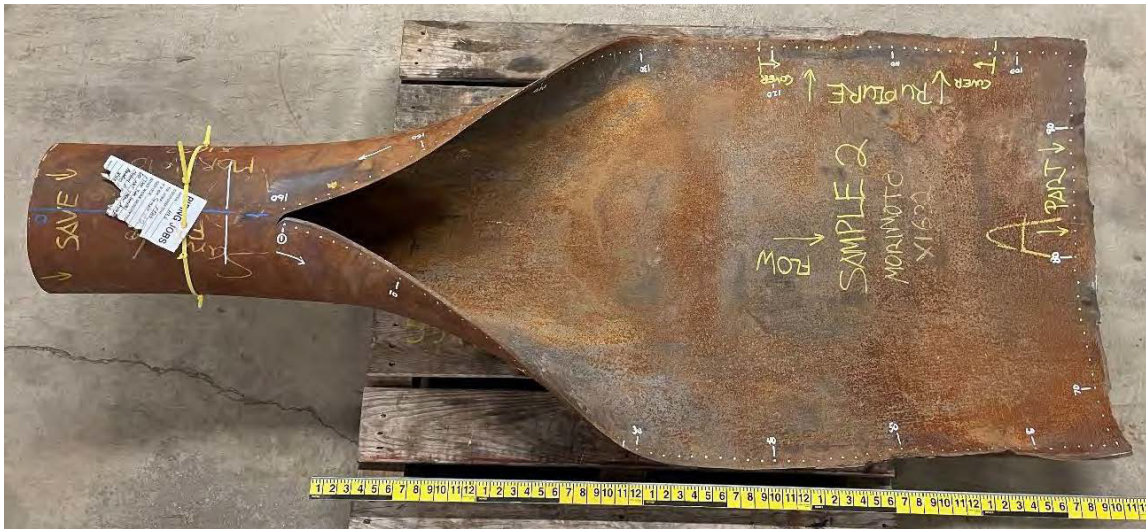
Figure 11. Ruptured tube. (Credit: PBF Energy)
