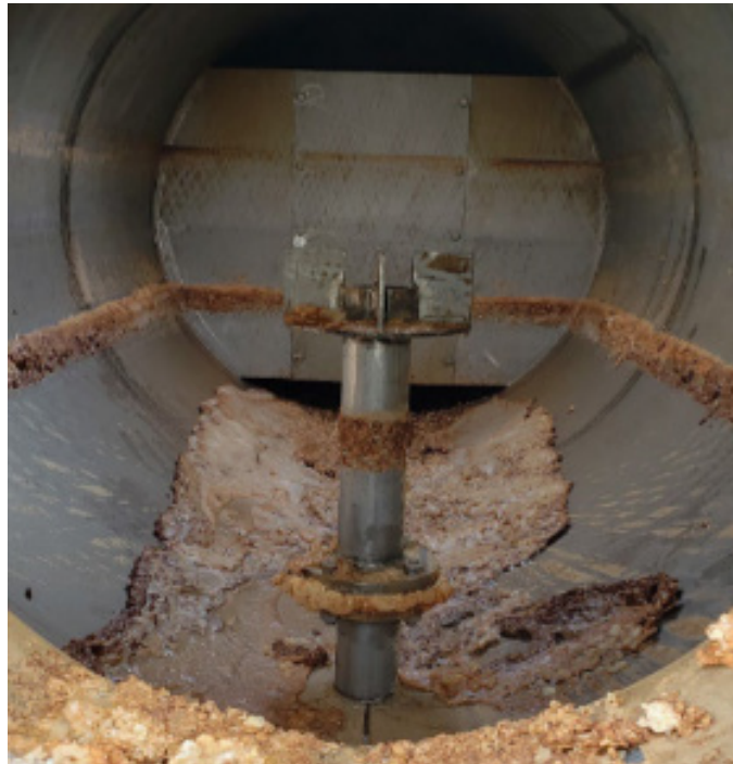
Figure 1. Tank Containing Solids at SABIC. (Credit: SABIC)
