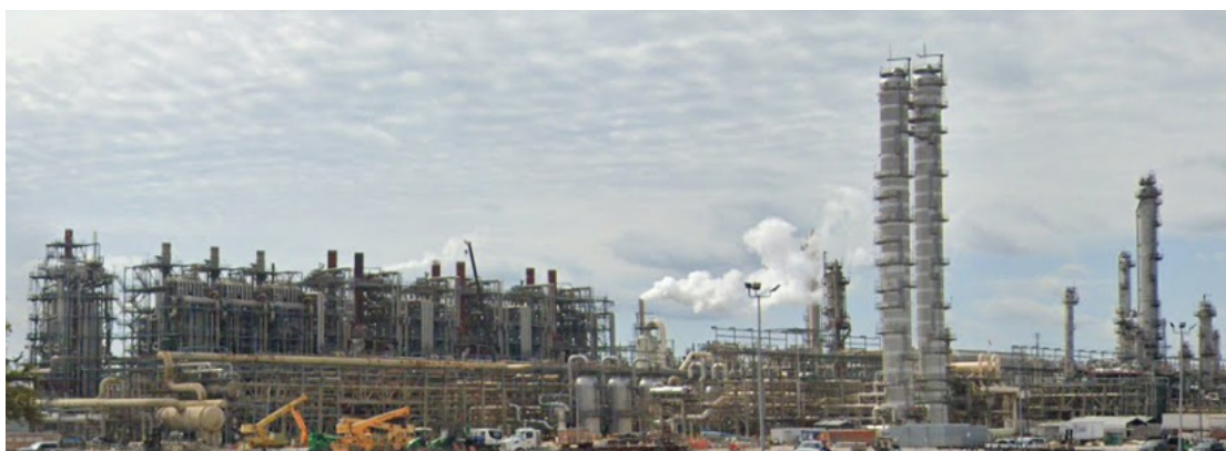
Figure 4. The Chevron Phillips facility in Sweeny, Texas. (Credit: Google Maps)
