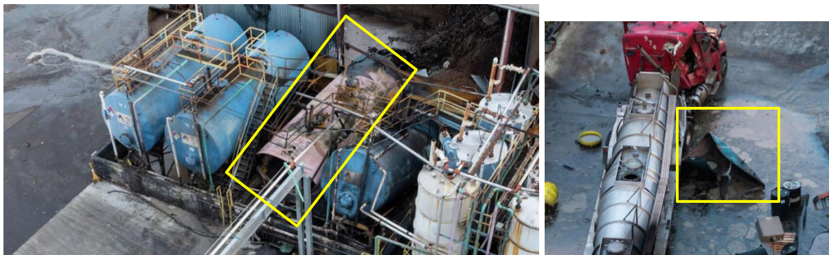
Figure 1. The tank that exploded (left). A portion of the tank after the explosion (right) (Credit: Tradebe, annotated by the CSB).
