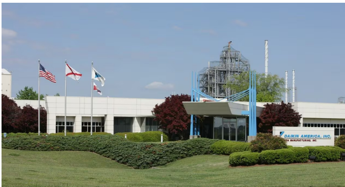
Figure 1. Daikin Facility. (Credit: al.com)
