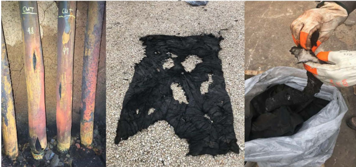
Figure 17. Failed fired heater tubes (left) and debris removed post-incident (center and right). (Credit: ExxonMobil)
