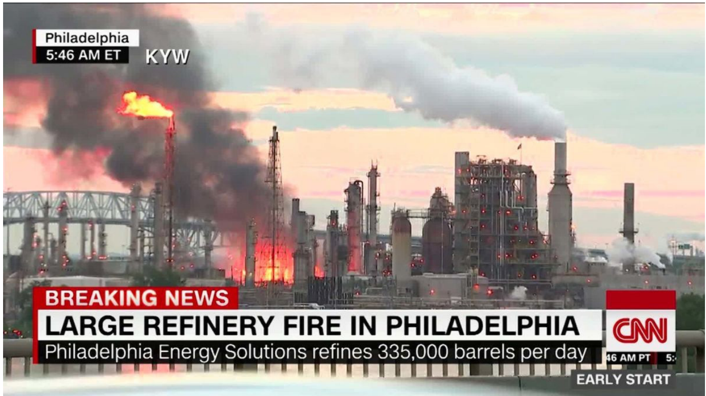
Figure 13. Photo of fire erupting at the PES refinery. (Credit: CNN).
