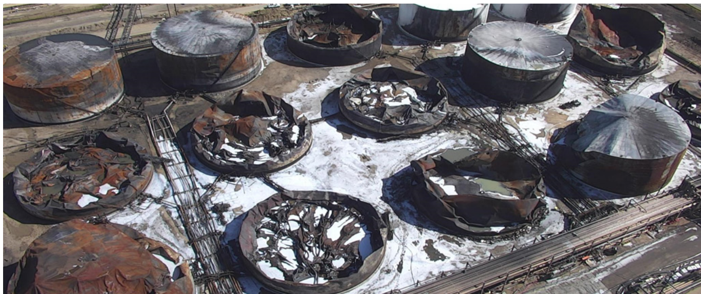
Figure 8. Photo included in the CSB ITC Investigation Report. This photo shows an overhead view of the First & Second 80's tank farm containment wall failure that allowed materials to enter the surrounding waterways on Friday, March 22, 2019. (Credit: ITC).
