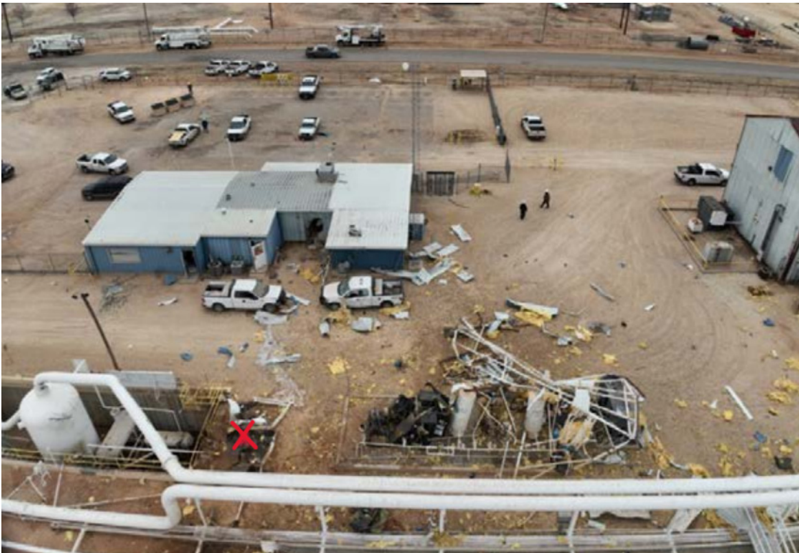
Figure 1. Aftermath of vessel overpressure, vessel location marked with red 'X.' (Credit: Kinder Morgan, annotated by CSB)
