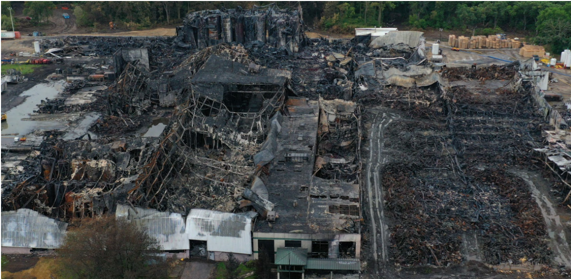
Figure 1. Damages After the Fire at Chemtool. (Credit: Chemtool)
