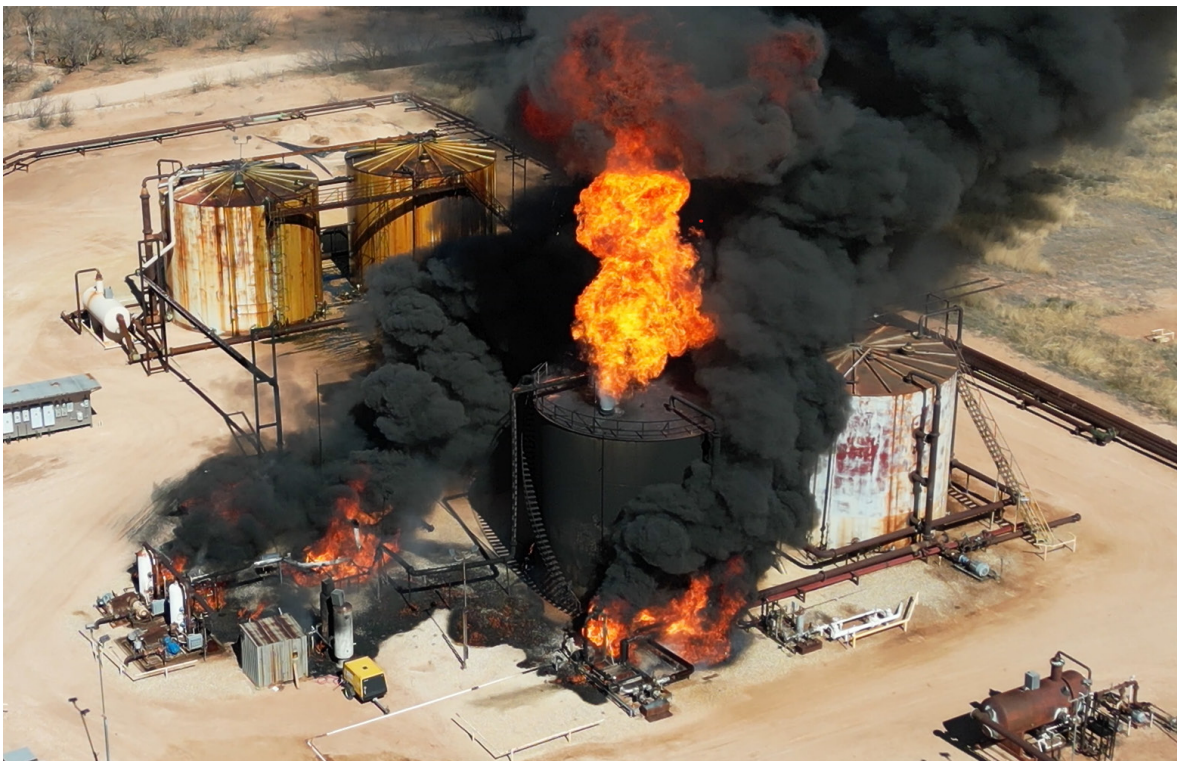
Figure 1. Aerial view of the fire and equipment involved in the incident. (Credit: Kinder Morgan)
