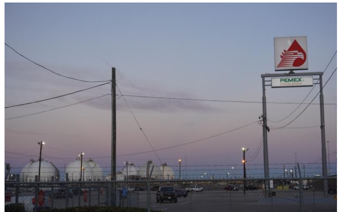
Figure 1. PEMEX Deer Park Refinery (Credit: CSB)
