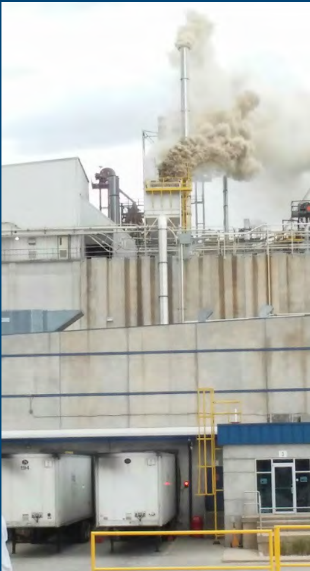
Figure 14. Image taken by a Didion worker of the May 29, 2017 fire. The structure on the roof of the building emitting smoke is a dust collector.
