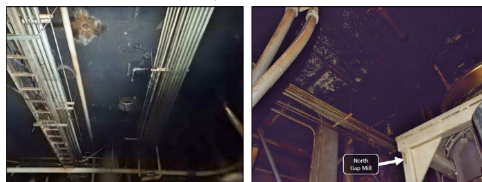
Figure 13. Example of overhead horizontal surfaces in 1B near the gap mill.
