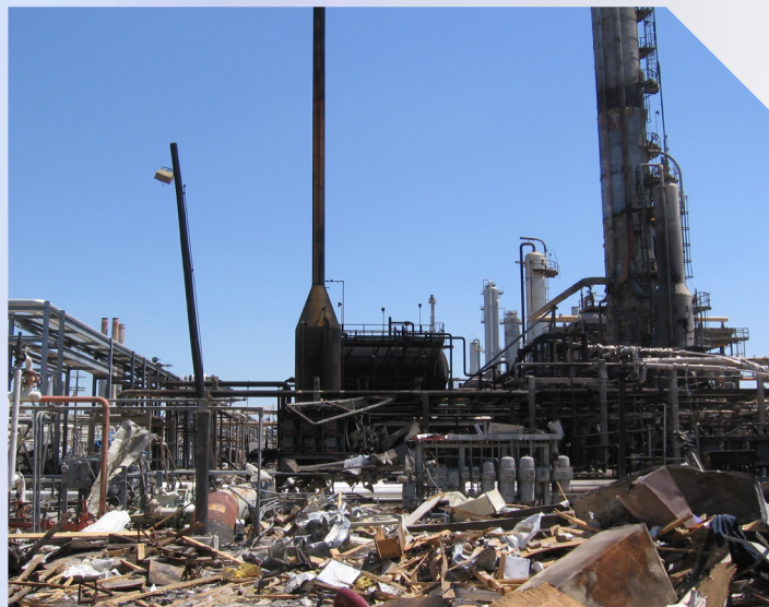
View of the BP Texas City refinery following the March 23, 2005 explosions and fire.
