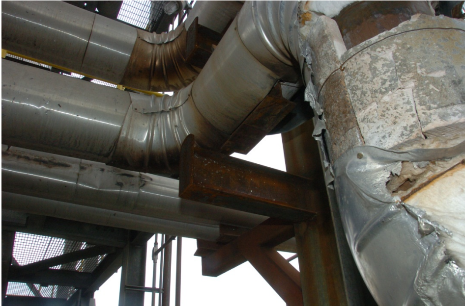
Figure 18. Pipe support location.
