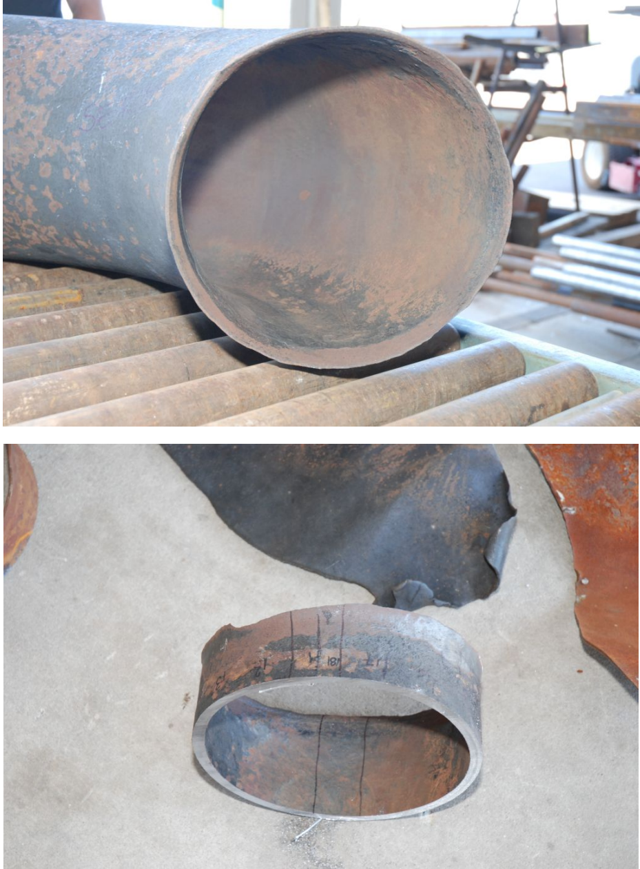
Figure 28. The fractured end of SER 34, before and after sectioning in August 2010.
