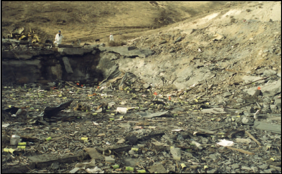
Figure 8. Booster Room 2 After Explosion
