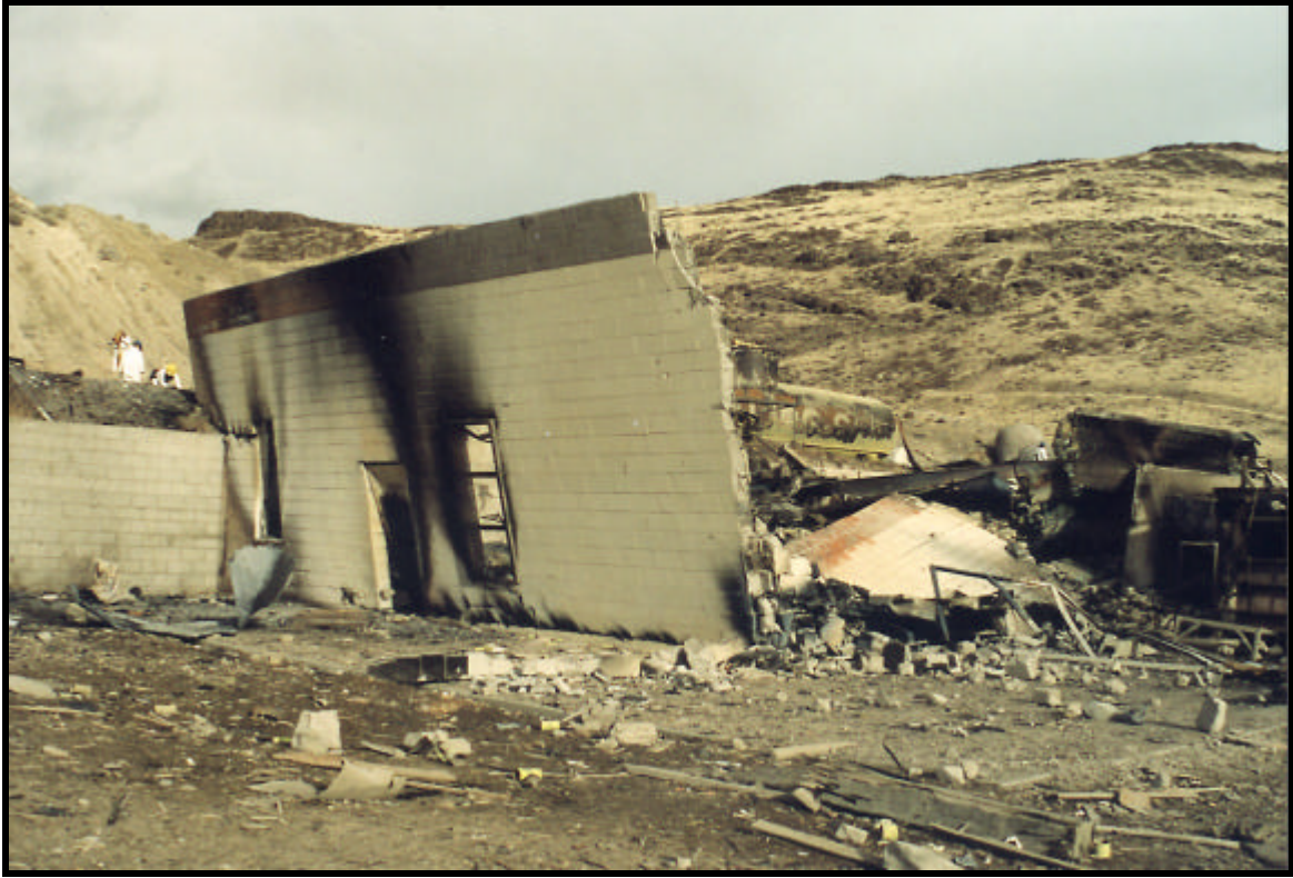
Figure 7. Booster Room 1 After Explosion
