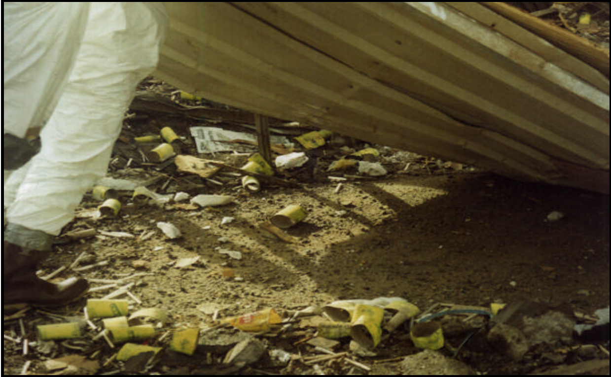
Figure 9. Lifting the Sliding Door
