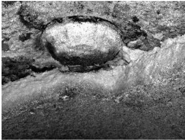
Figure 7. Polymer plugging the polymer catch tank vent nozzle.
