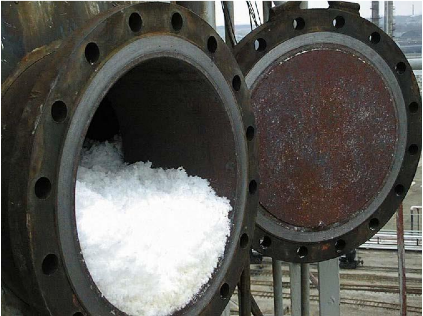
Figure 9. Popcorn polymer in a manhole from another undisclosed butadiene unit, published in the Butadiene Popcorn Polymer Resource Book. (Credit: International Institute of Synthetic Rubber Producers Inc. [12, p. 261])
