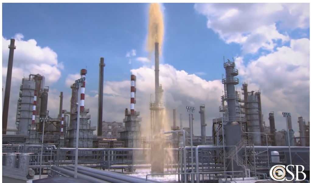
Figure 7. Image from the CSB's animation of the BP Texas City explosion.
