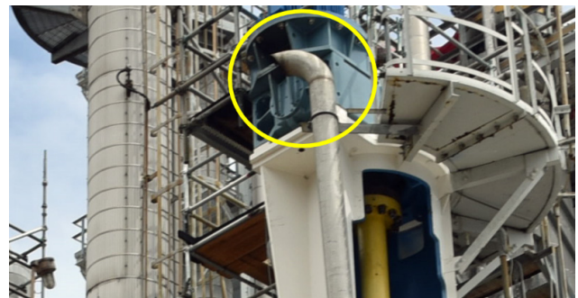
Figure 2. Horizontally-aimed piping from Kuraray's emergency pressure-relief system.
